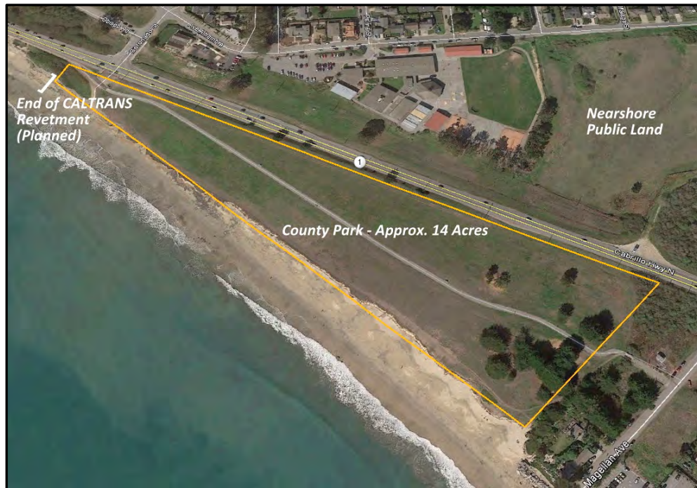
Figure 7: Aerial View of Public Parkland
